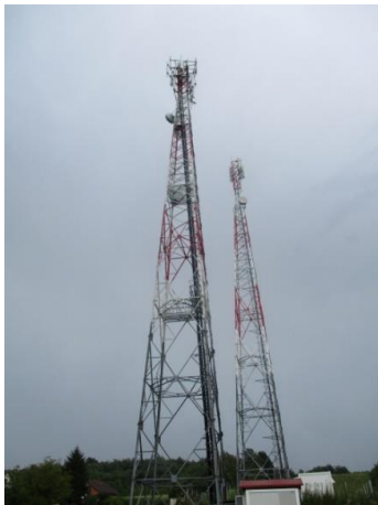
Figure 2. Collocated HF EMF sources installed on two masts comprised of following systems: FM, TV, LTE 800, GSM 900, UMTS 900, LTE 1800, LTE 1800, UMTS 2100
